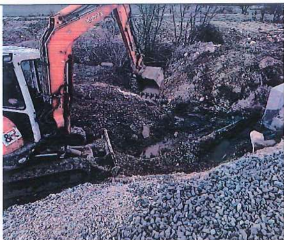
T6 North side – Filling collapsed section
