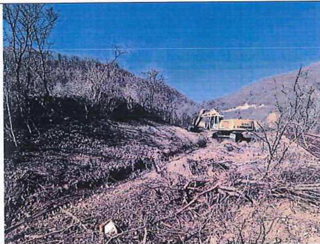
Clearing and grubbing in Kacanik Station
