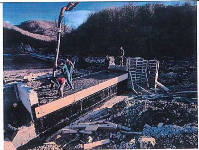
Construction RHS and LHS ditches in area after Ferizaj
