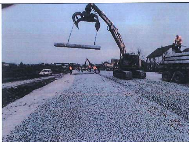
Laying of new rails and installation of turnouts
