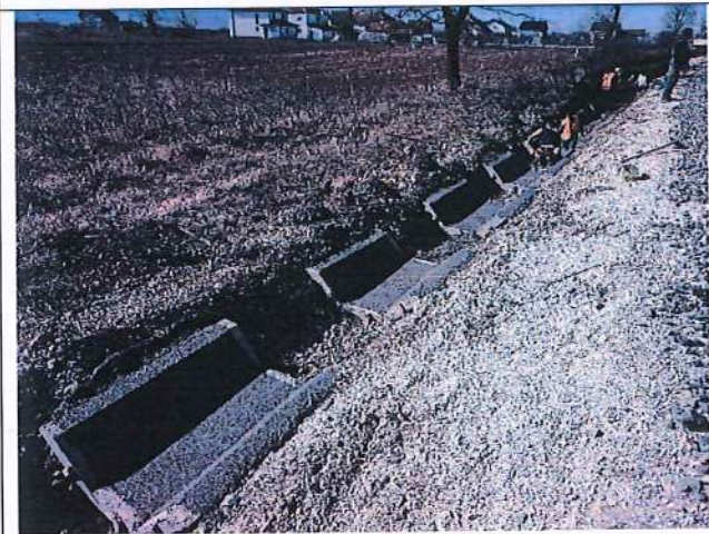
Construction of subdrain channel in Lypjan
