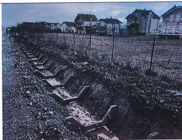
Construction of subdrain channels in Stagove area
