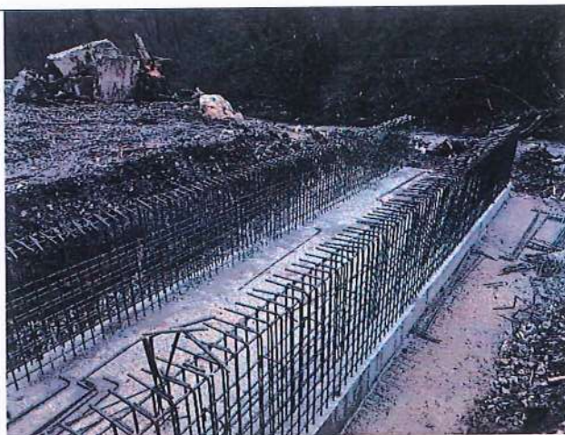
Constructed culvert body
