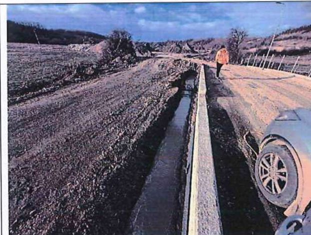
Construction and testion of sil improvement with sand&gravel mixture
