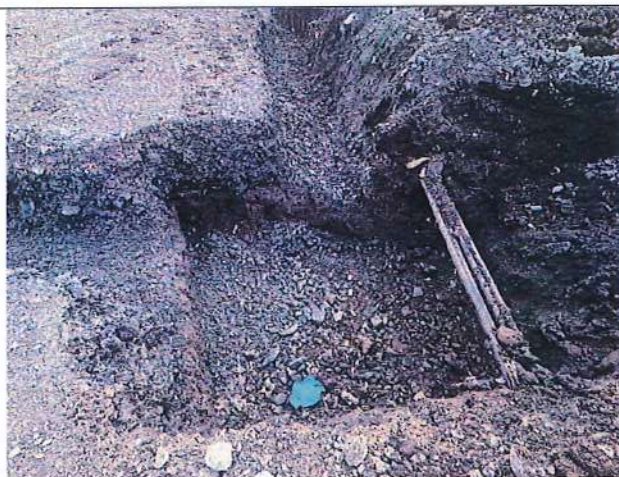
T7 south portal
