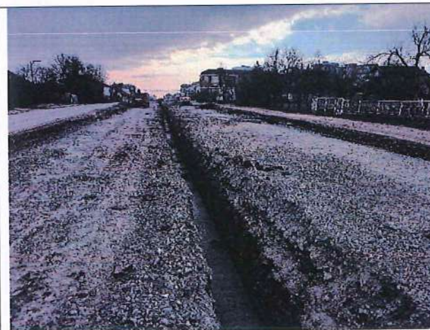
Construction of RHS and LHS ditches in Lypjan Station ch. 262+200 – 262+282
