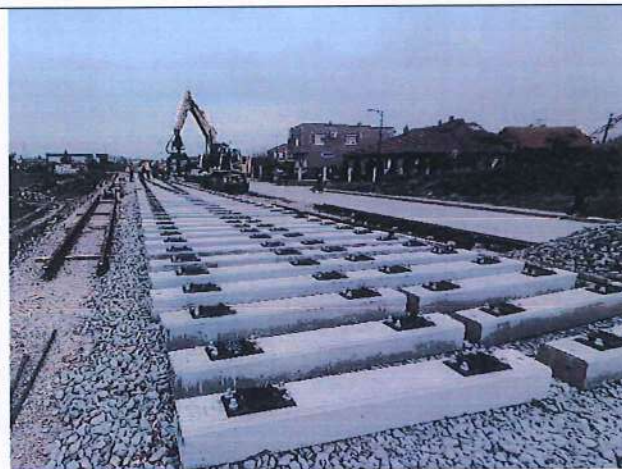
Laying of new rails and installation of turnouts
