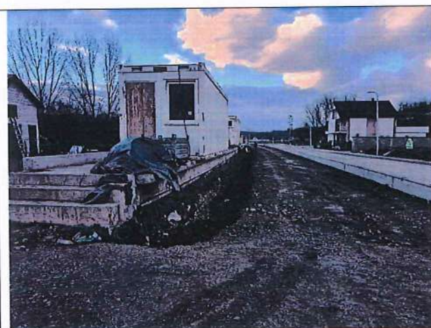
Construction and testion of sil improvement with sand&gravel mixture
