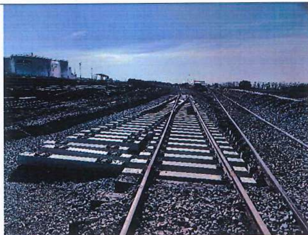
Laying of new rails and installation of turnouts
