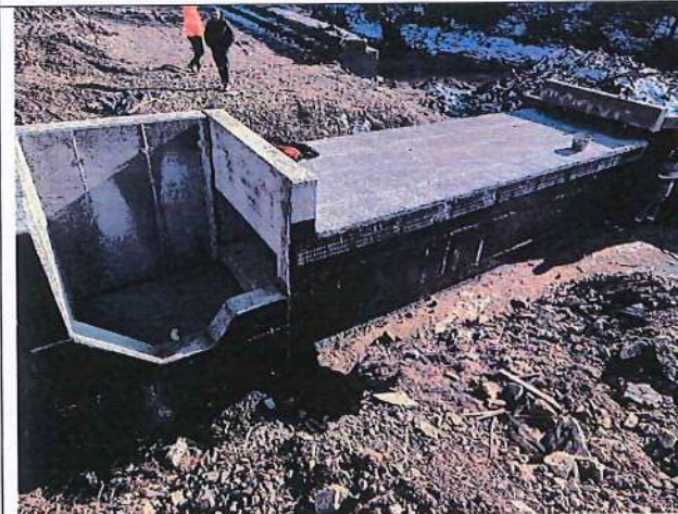
Installation of waterproofing and protective concrete
