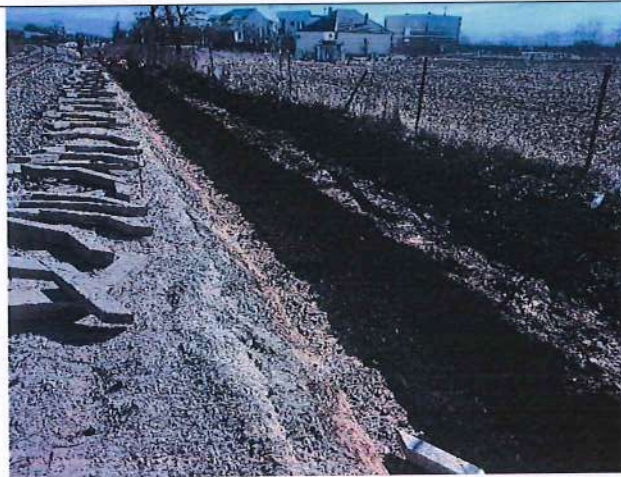
Construction of subdrain channel in Lypjan
