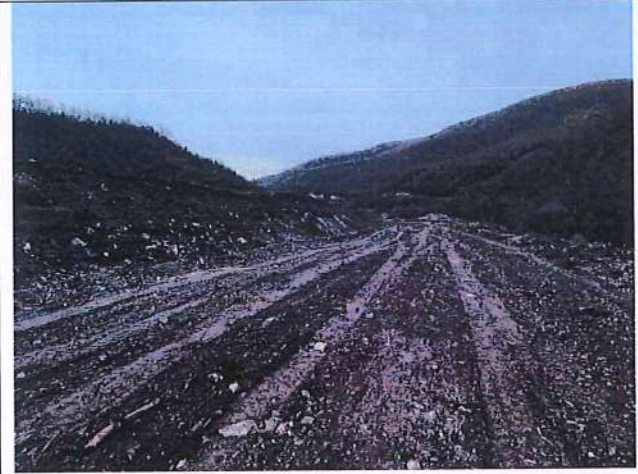
Clearing and grubbing ch. 284+160 – 284+400
