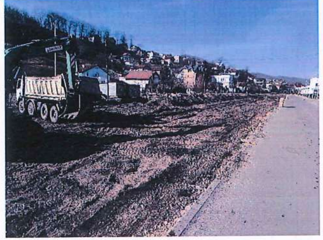
Clearing and grubbing in Stagove area from ch. 296+500 – 297+000.
