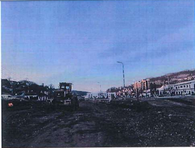
Clearing and grubbing in Stagove area from ch. 296+500 – 297+000.
