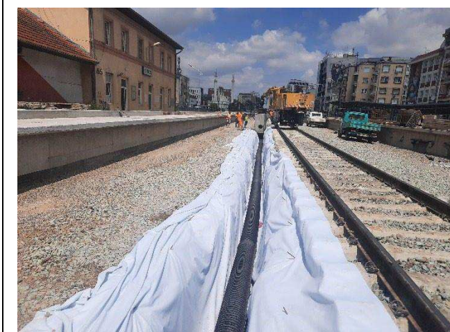
Laying of the preforated pipes and geotextile
