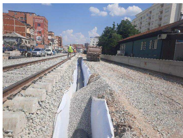
Filling with filter gravel material
