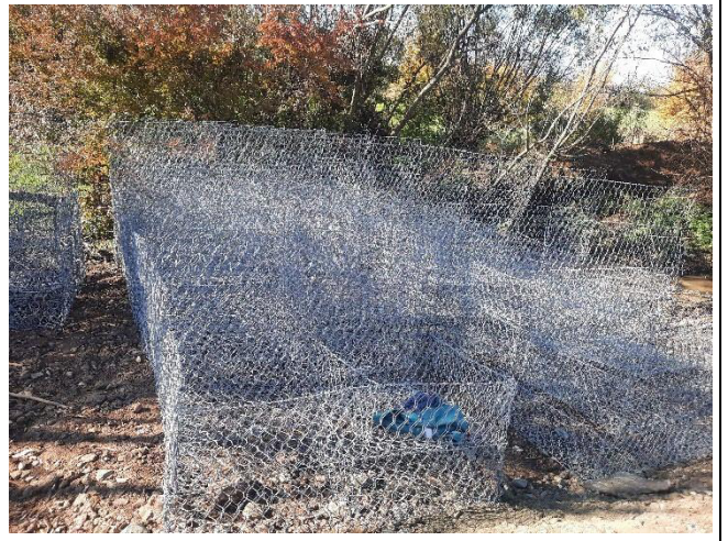
Filling of gabion cages with quarry stones
