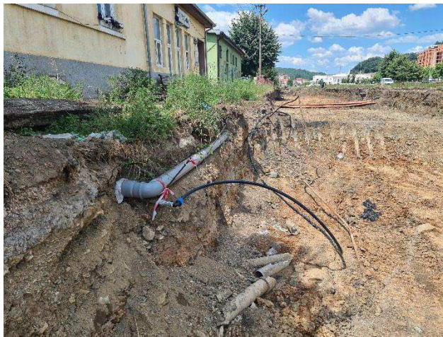
Sewerage old pipe cs 1666+10m
