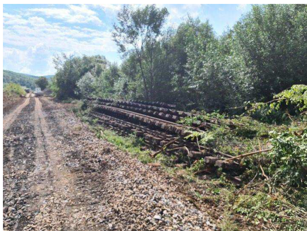
Dismantling of existing railway S49 on wooden sleepers, Metalurgjia
