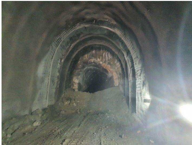
Additional support measures in tunnel 6 (North part)
