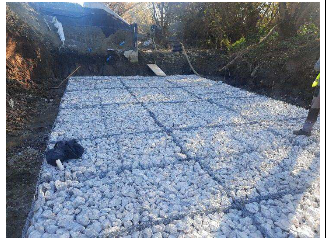
Filling of gabion cages with quarry stones
