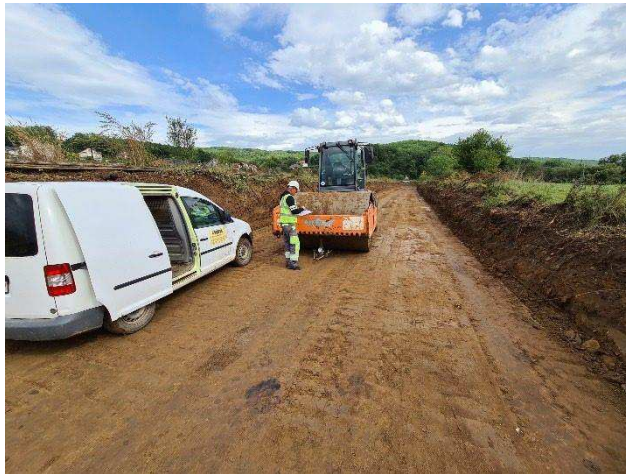
Excavation and testing of natural ground Metalurgjia area
