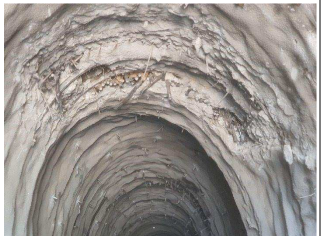
Geometry correction of the temporary lining, Tunnel 7
