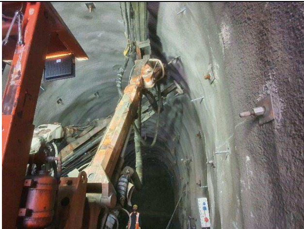
Installation of radial bolts Ch: 307+110.75 – 307+150.8
