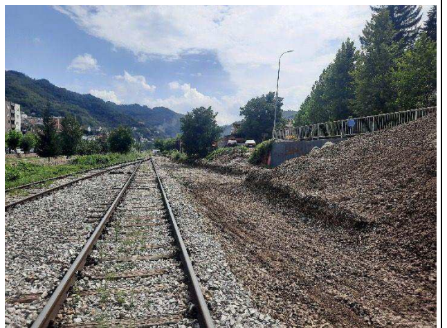
Dismantling of existing railway S49 on wooden sleepers, Stagove area
