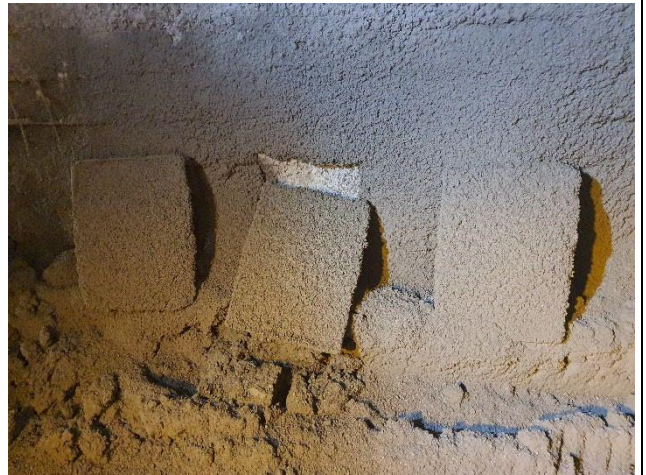
Additional support measures in tunnel 6 (North part)
