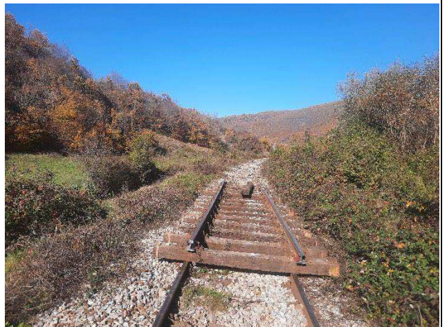
Dismantling of existing railway S49 on wooden sleepers, Stagove area
