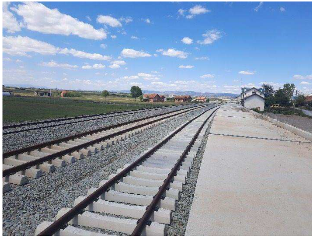
Assembling and mounting of turnouts
