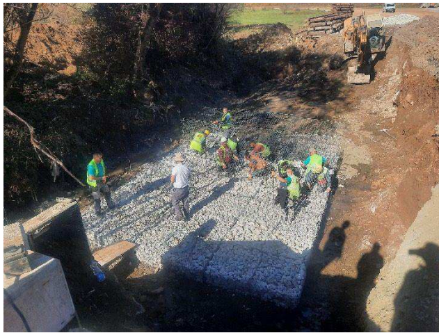
Filling of gabion cages with quarry stones
