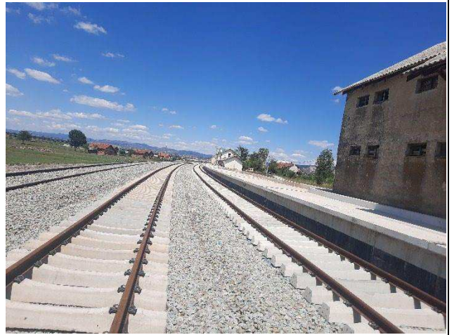
Removal of the old ballast Kacanik Station
