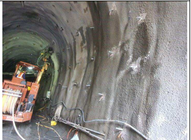
Installation of radial bolts Ch: 307+110.75 – 307+150.8
