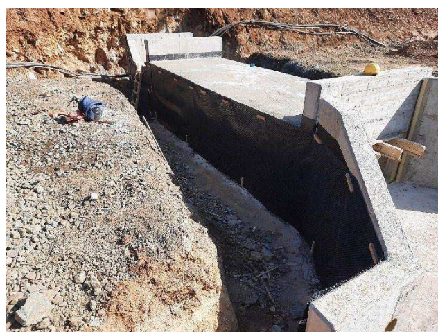
Filling with filter gravel material
