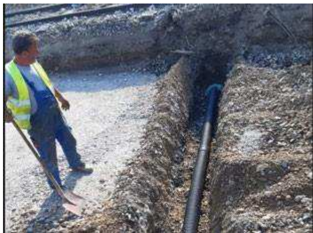
Crossing pipes for future in Hani I Elezit Station
