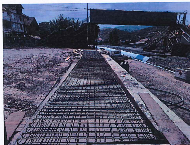
Installation of reinforcement in Platform
