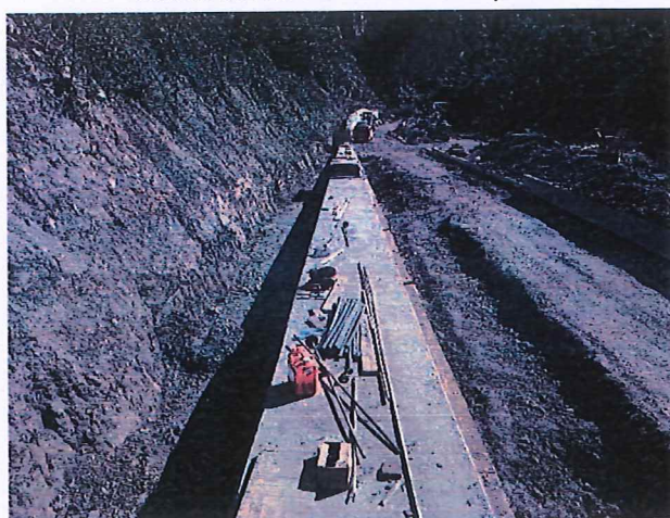
Constructed wall above the piles
