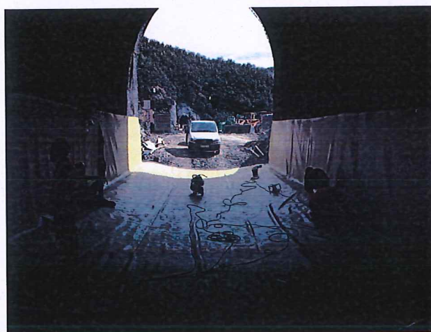
Installation of membrane in seg.36 & 37
