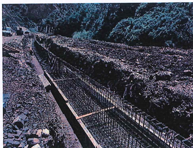
Installation of reinforcement RW_36 Right
