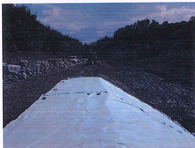
Geotextile under the rip rap before T1
