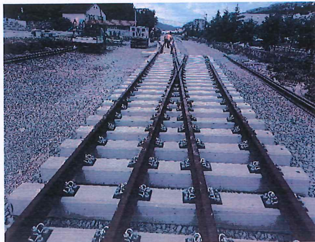
Assembly and mounting of turnout
