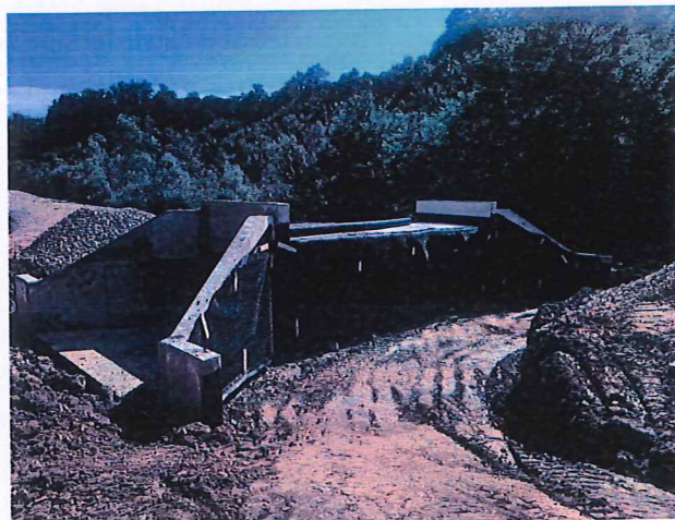
Construction of the line in Kacanik Station
