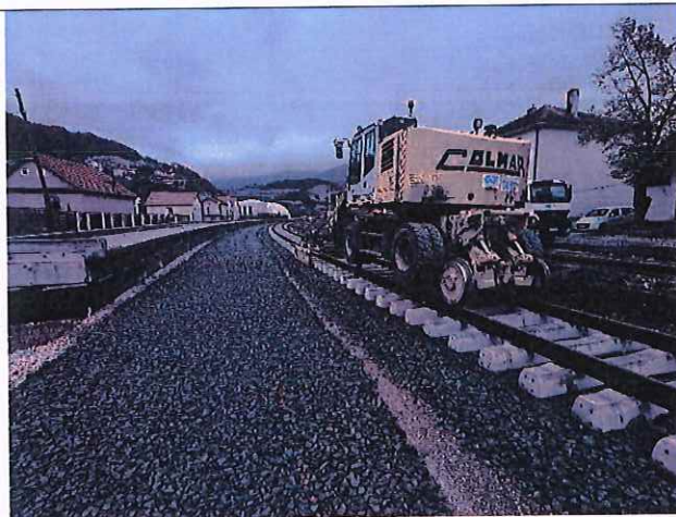
Laying of new rails UIC 60 EI and S 49
