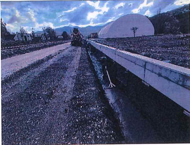
Installation of perforated pipes, geotextile and filter gravel material
