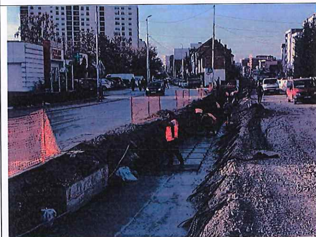
Constructed wall 14_Left
