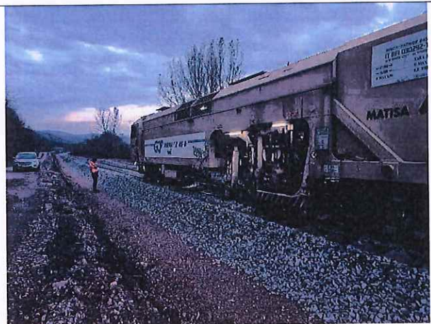
Laying of first layer of ballast and new concrete sleepers
