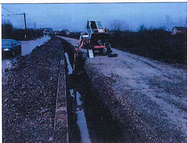
Excavation of the channel
