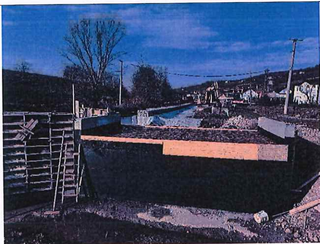
Construction of side ditches in the section Ferizaj ch. 282+650 - 283+086
