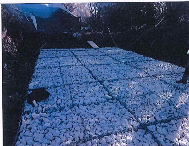
Filling of gabion cages with quarry stones
