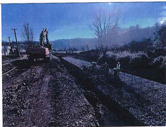
Constructed Gabions
