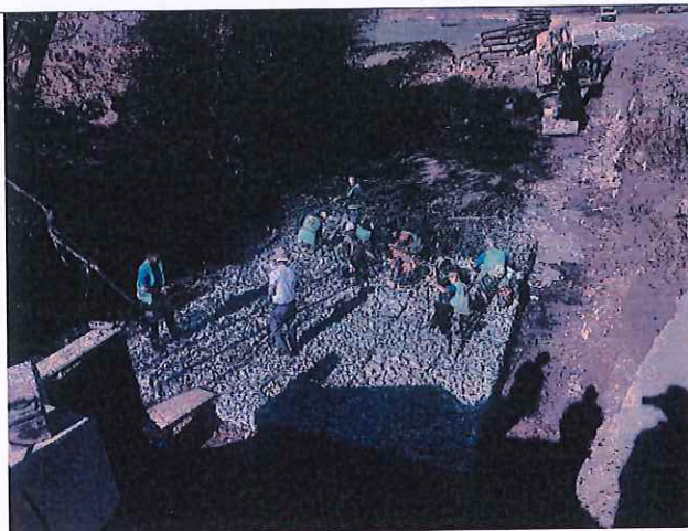
Filling of gabion cages with quarry stones
