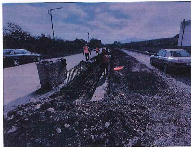
Constructed walls 19_Right
