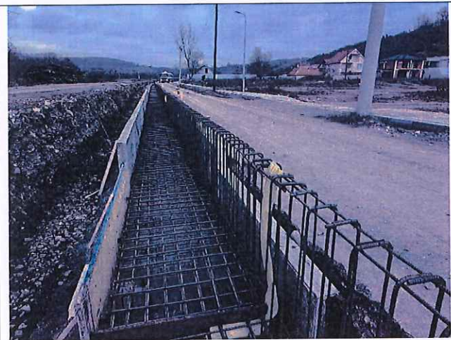
Construction of retaining walls RW-19 Left and RW 20 Left in Stagove
