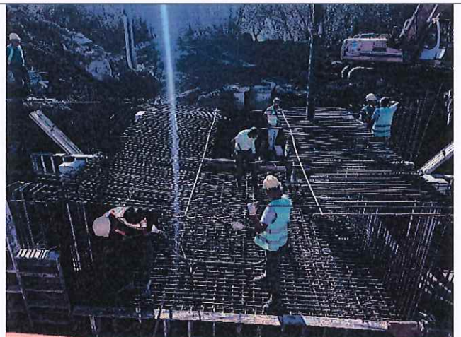
Pouring of concrete for foundation
