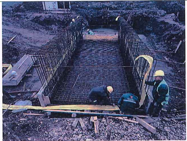
Construction of side ditches in the section Kusine - Ferizaj
