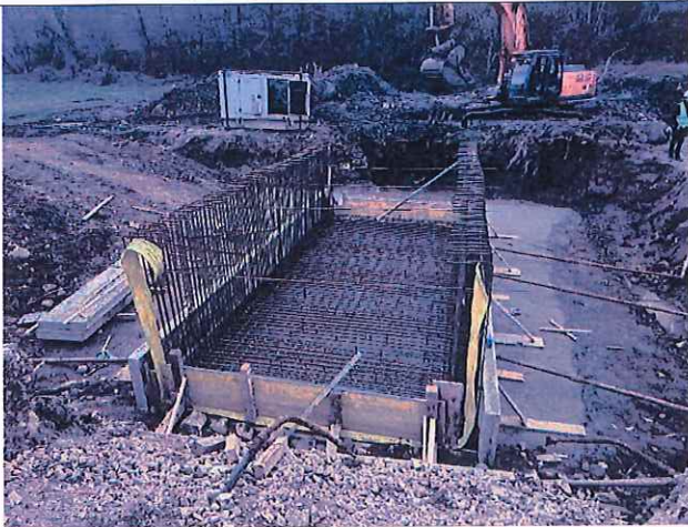
Construction of side ditches in the section Kusine - Ferizaj
