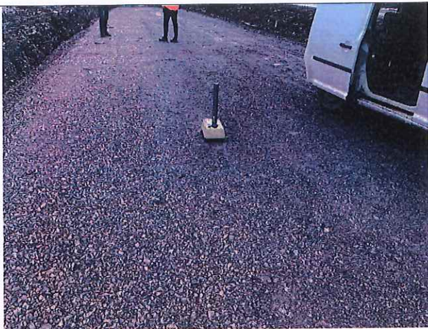
Construction of upper protective layer in Fushe Kosova cs 133+7.5-cs 136
