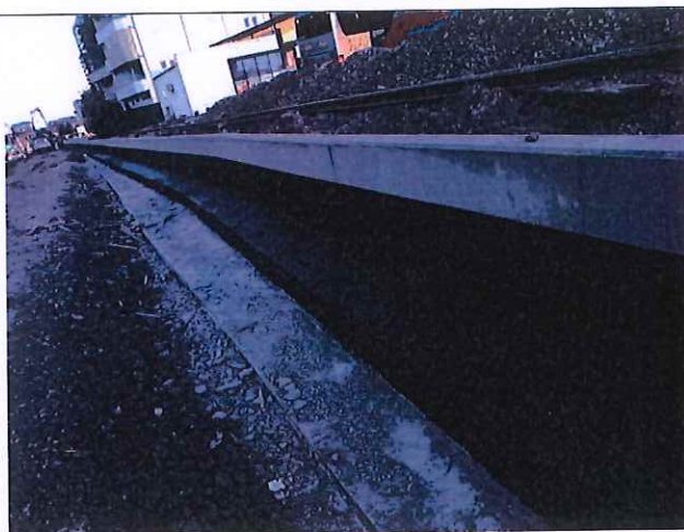
Constructed wall 18_Right
