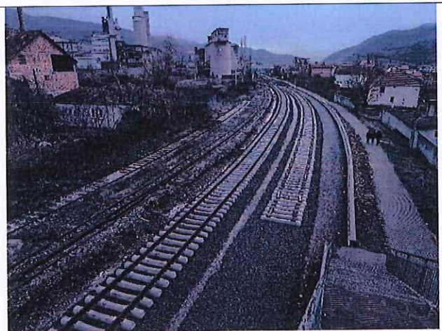
Laying of new rails UIC 60 EI and S 49
