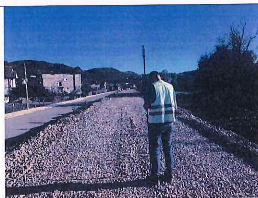
Inspection of the subgrade layer
