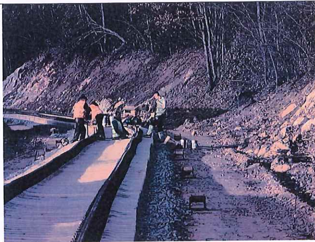
Laying of first layer of ballast and new concrete sleepers
