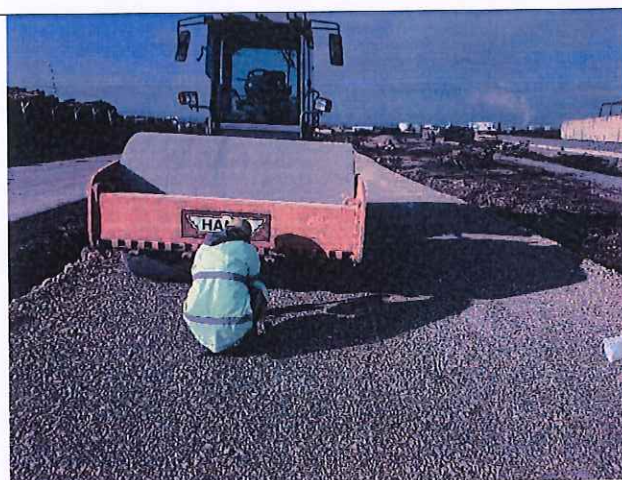
Construction and testing of the upper protective layer
