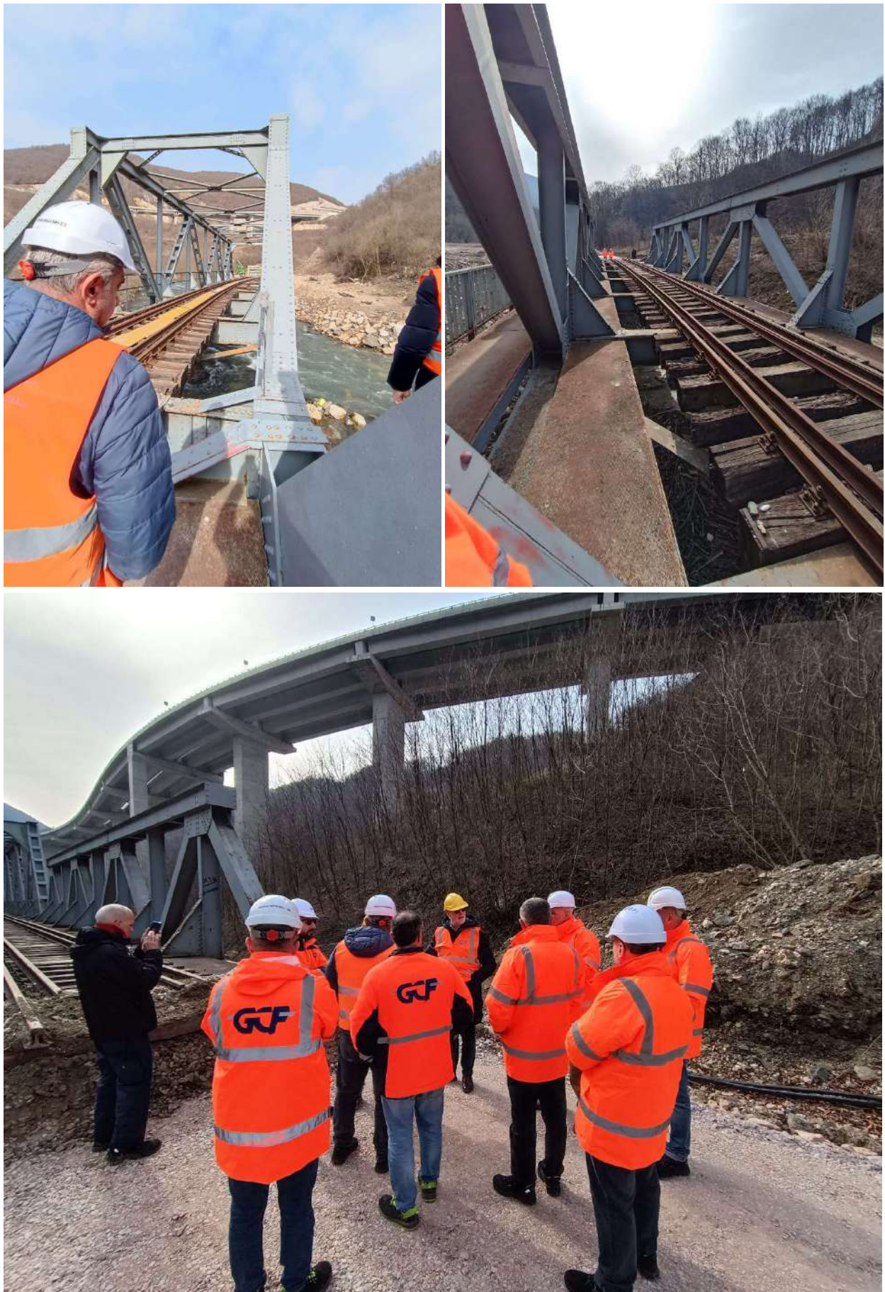
Visit of the bridges for Phase 1 Works
