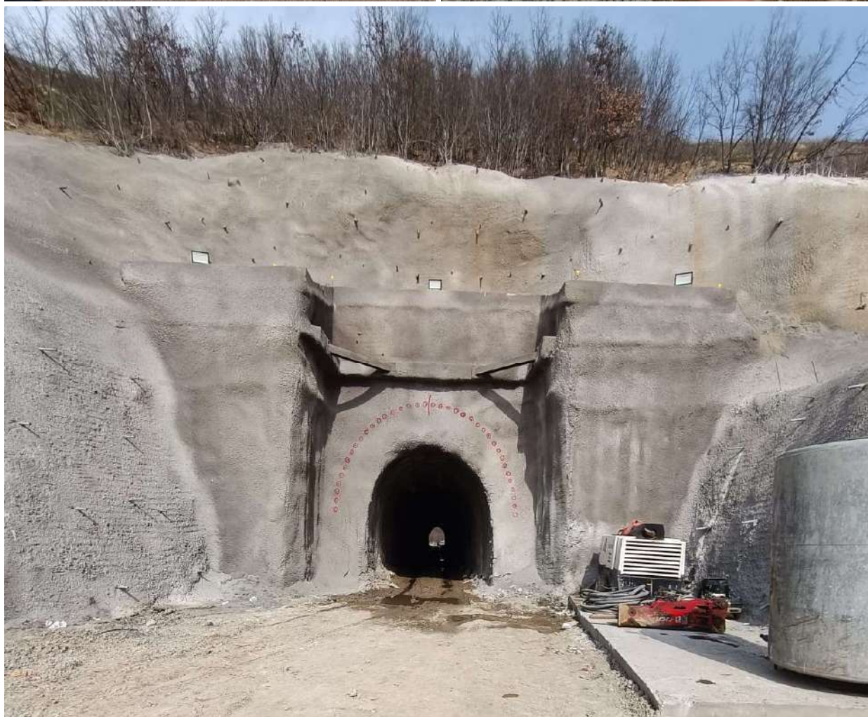
Visit of the tunnels under construction for Phase 1 Works
