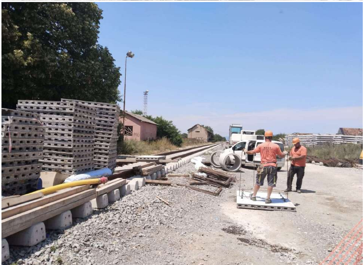
Ongoing R/C works near Mitrovicë and Prelluzhë
