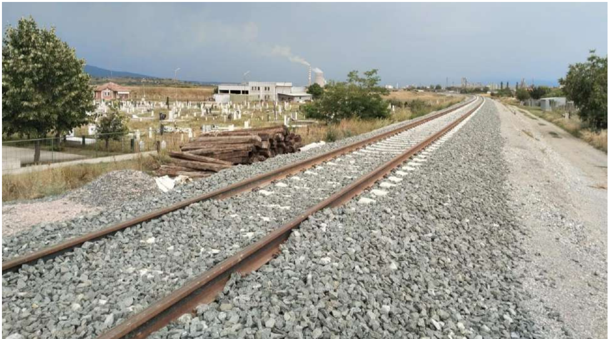
Figure 1 Current view of the line around Obiliq
