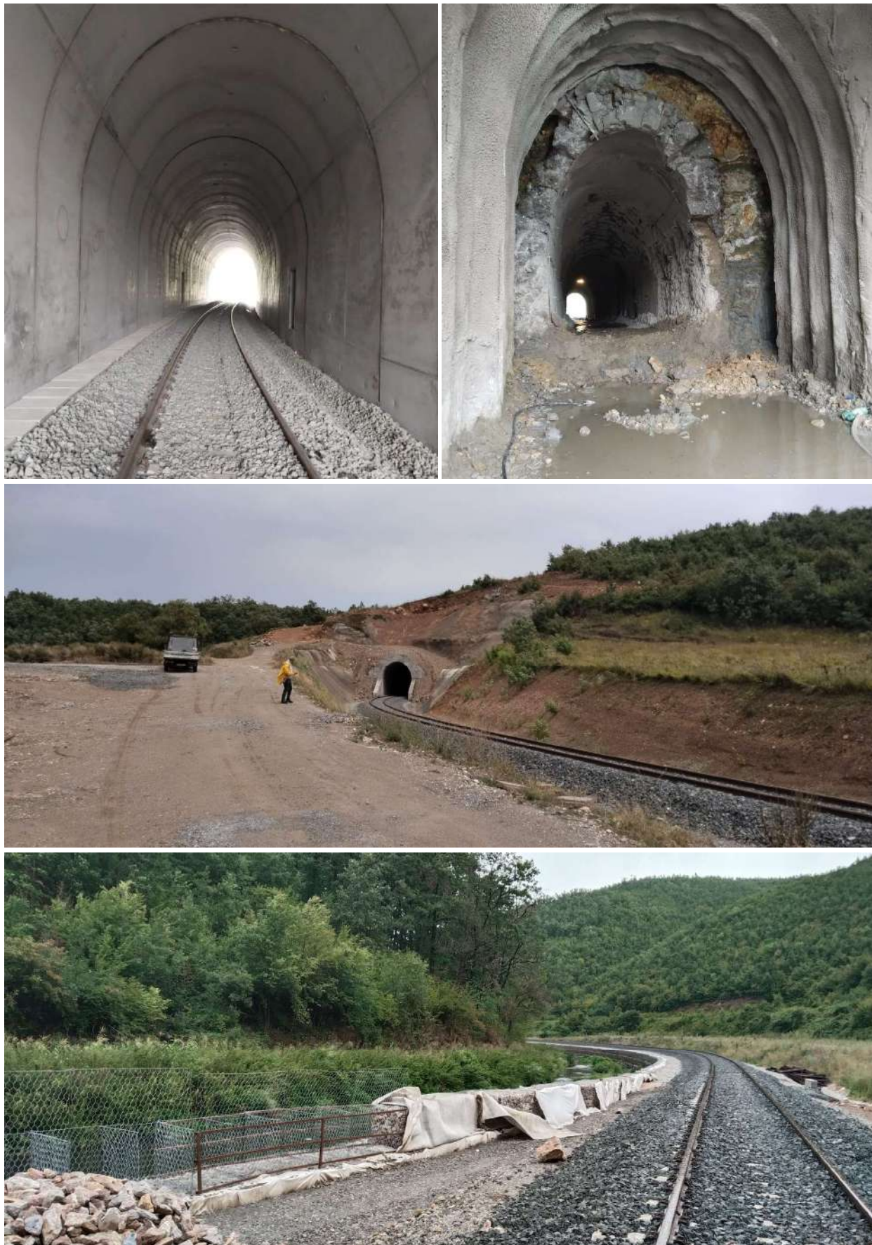
Ongoing construction for tunnels and railway track works
