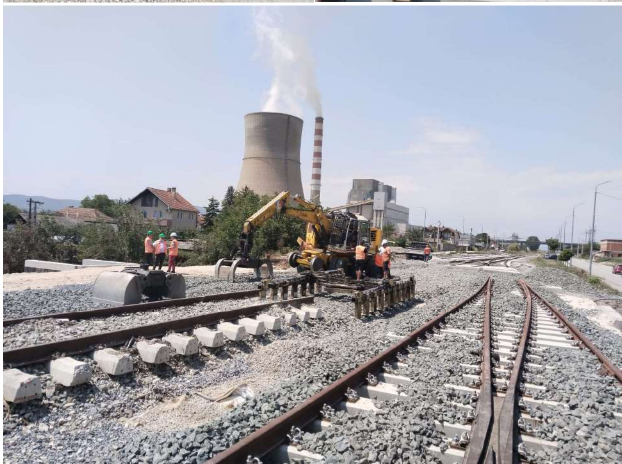
Ongoing track works near Kastriot
