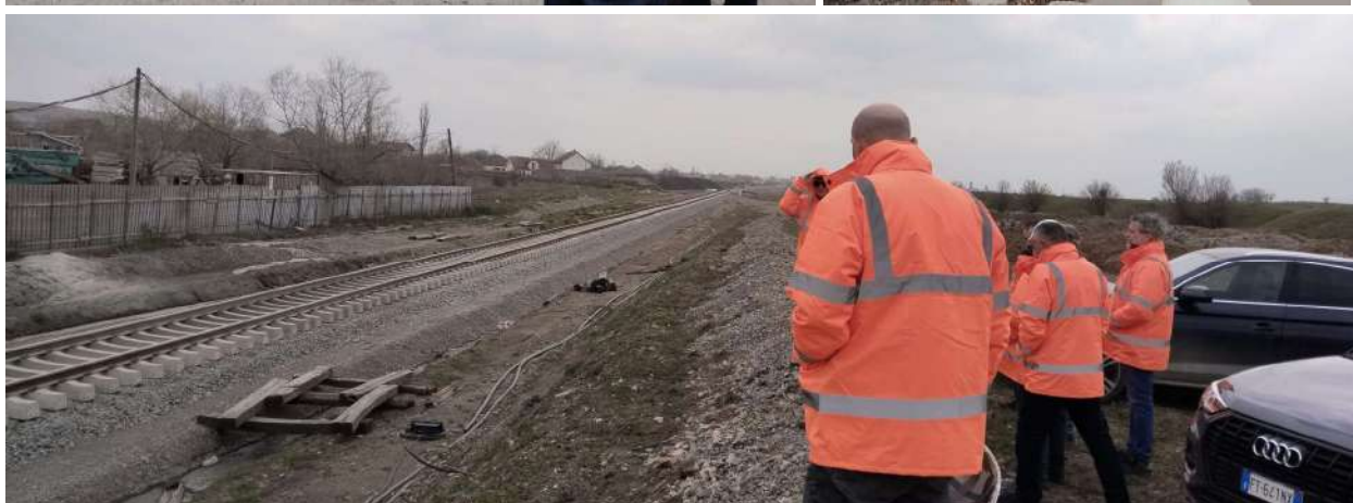
Visit of the trackworks overpass and culvert near Kastriot for Phase 2 Works
