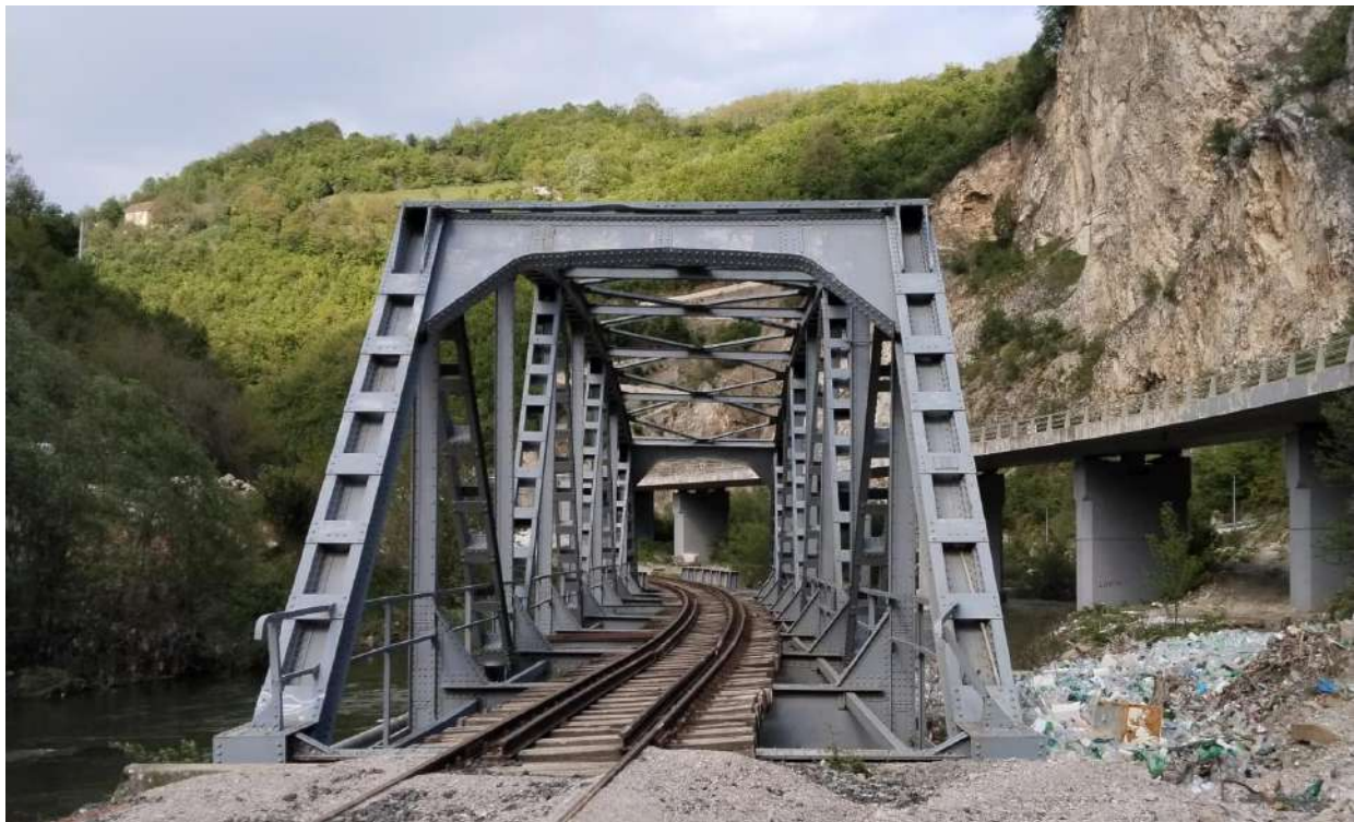
Figure 2 Steel Bridge near Kacanik
