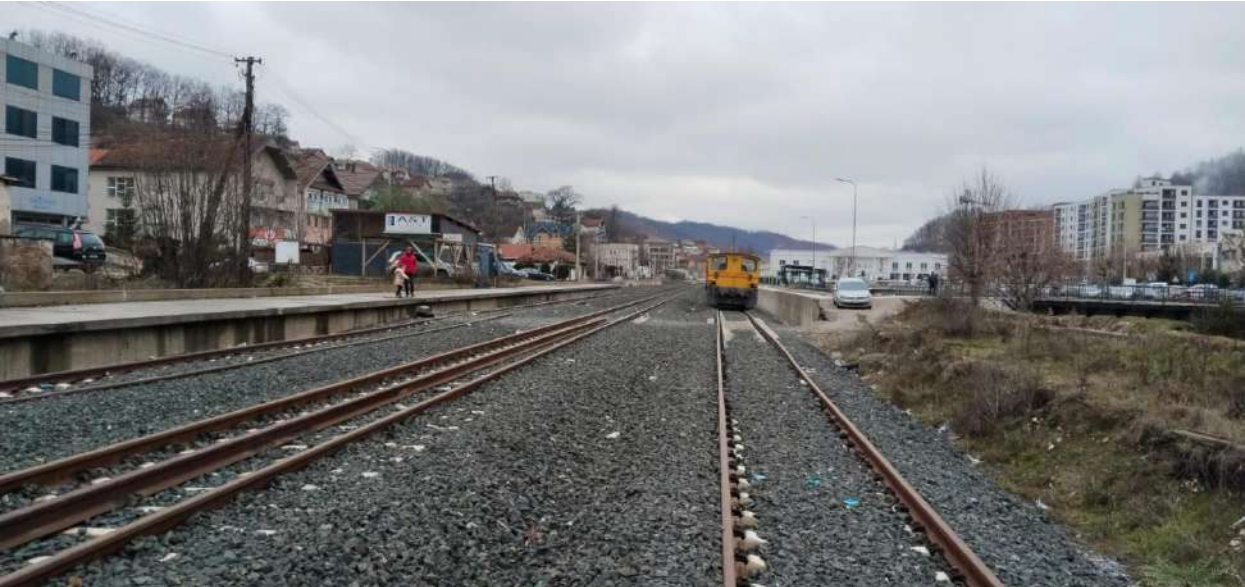
The Kacanik Station is located between PK 299+740.70 and PK 300+608.35.
