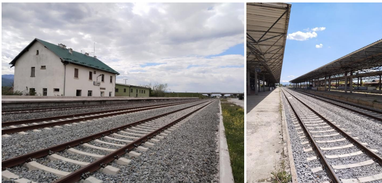
Figure 1 Operable section of the line between Gures and Fushë Kosovë
