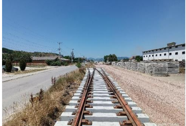
Turnouts have been delivered and temporary assembled near the Station Vushtrri and Mitrovica. (May 2025)
