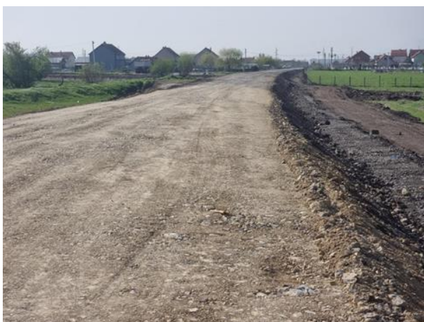
Filling Soil Improvement at seg. 1
