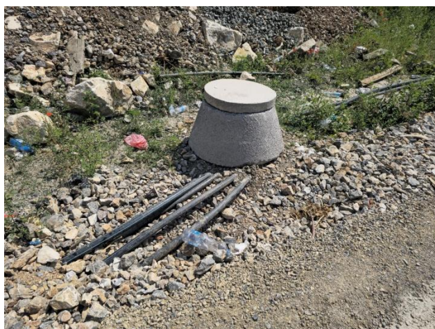
Bad practice. Optic Cables left exposed (June 2025)
