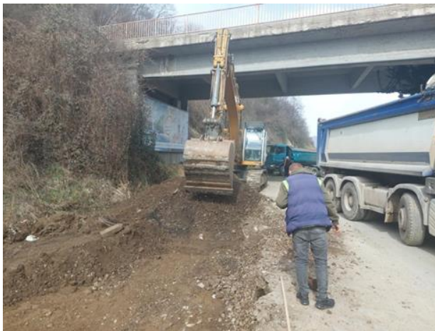
Removal of existing Ballast at seg. 32
