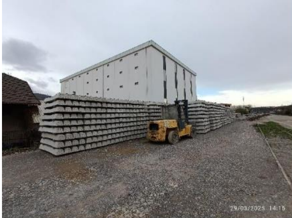
New Sleepers B70 2.60m and 2.40m stocked in Mitrovica Station (March 2025)
