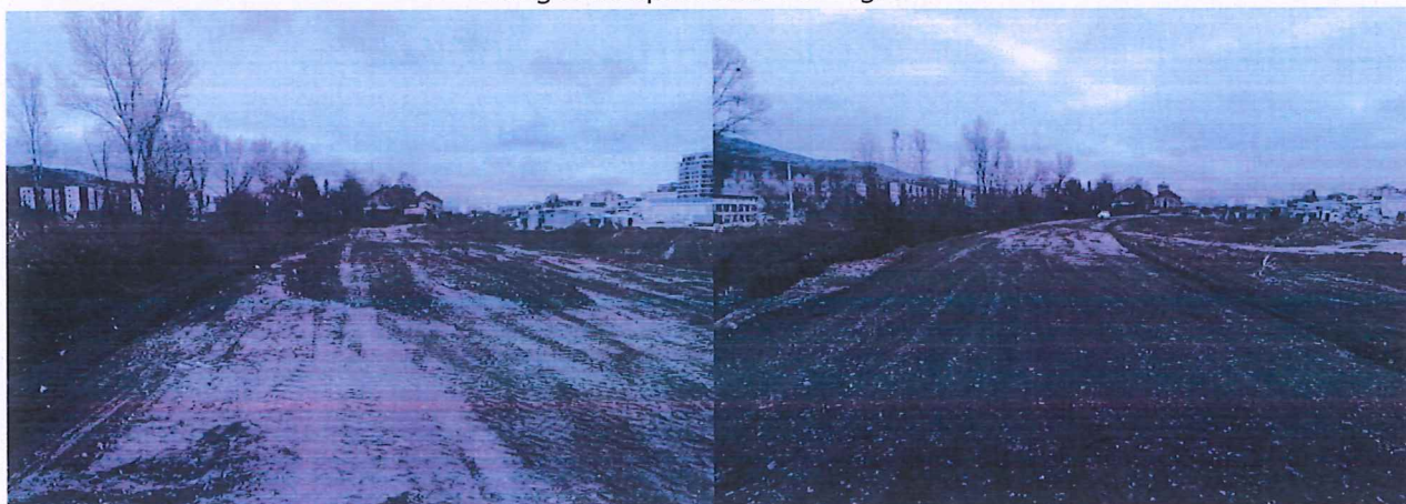
Filling soil Improvement at Seg. 35
