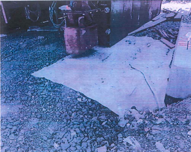
Good practice. Near br 26, slope excavated carefully without throwing material into river. (16 October 2024)
