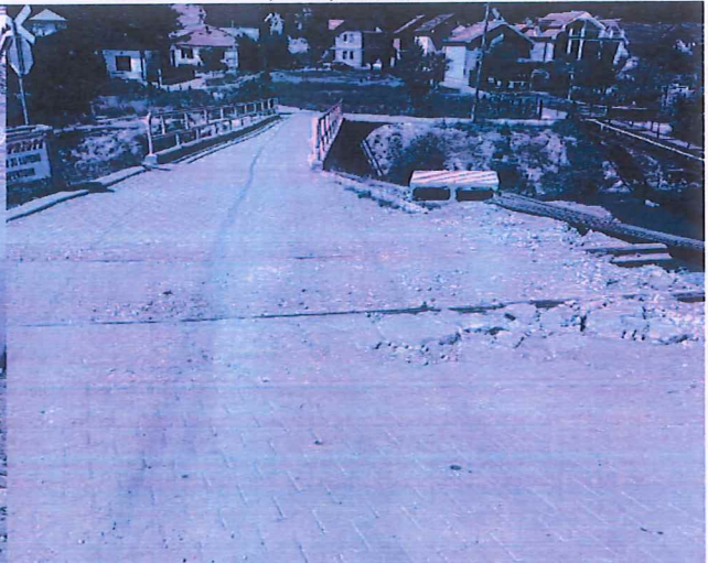
Bad practice, Access to br 24, Excessive material disposed in unapproved site. (16 October 2024)
