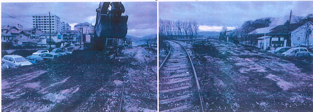
Removal of existing Ballast at Seg. 33
