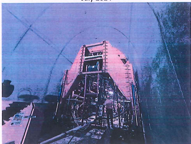
Good practice: Finnal lining, Tunnel T6 July 2024
