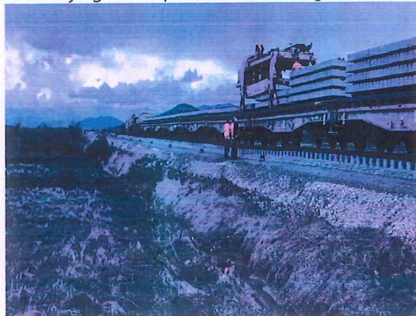
Laying of Sleepers and Rails – Segment 16
