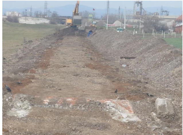
Removal of existing ballast seg. 2
