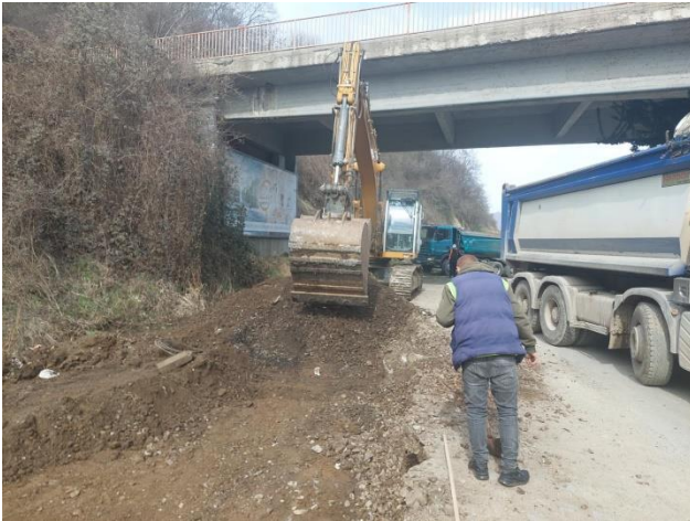
Removal of existing ballast seg. 32
