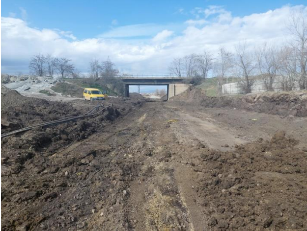
General Excavation seg. 2
