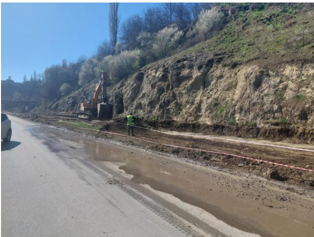
Removal of existing ballast seg. 32
