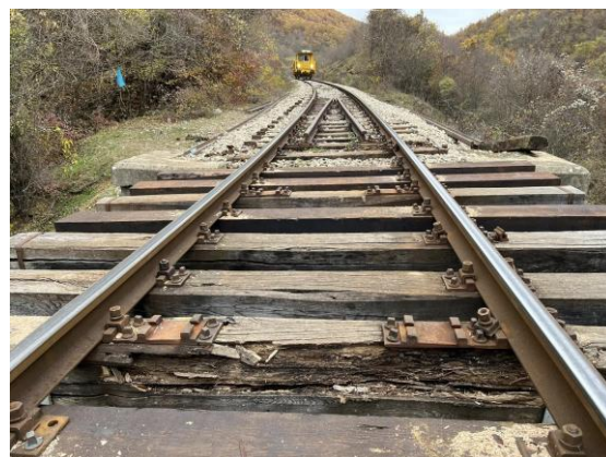
Before the works
