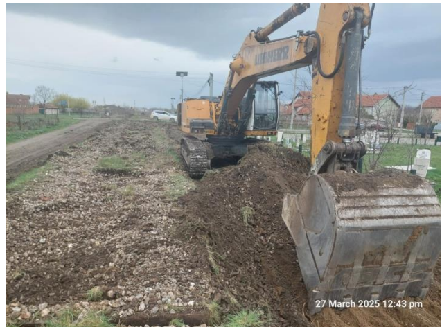
Removal of existing ballast seg. 1
