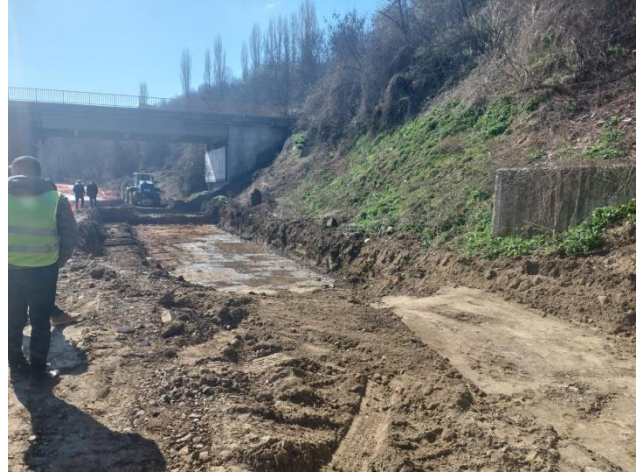
Excavation in Land Improvement seg. 32
